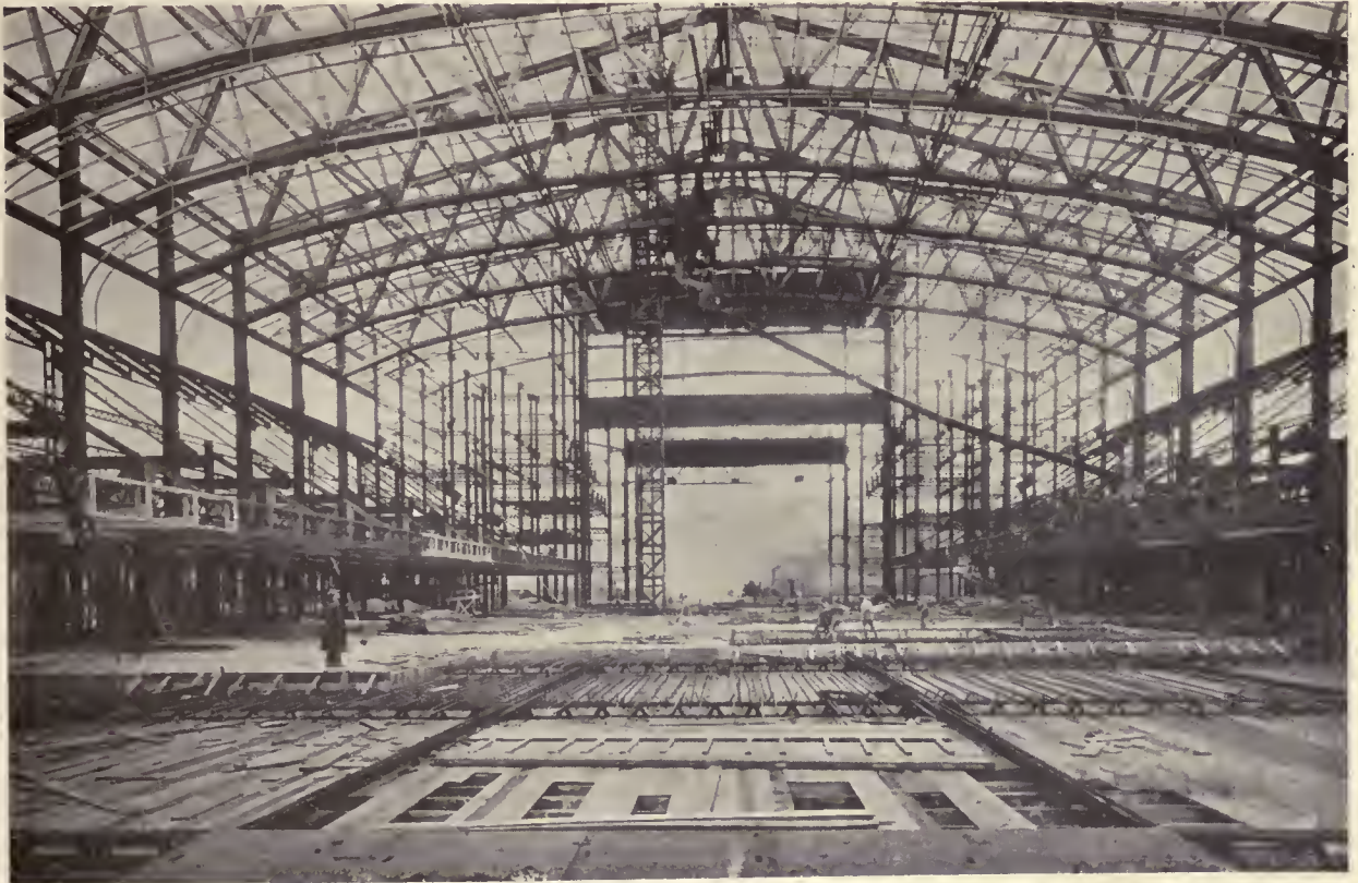
A VIEW FROM THE MAIN FLOOR DURING STEEL ERECTION
